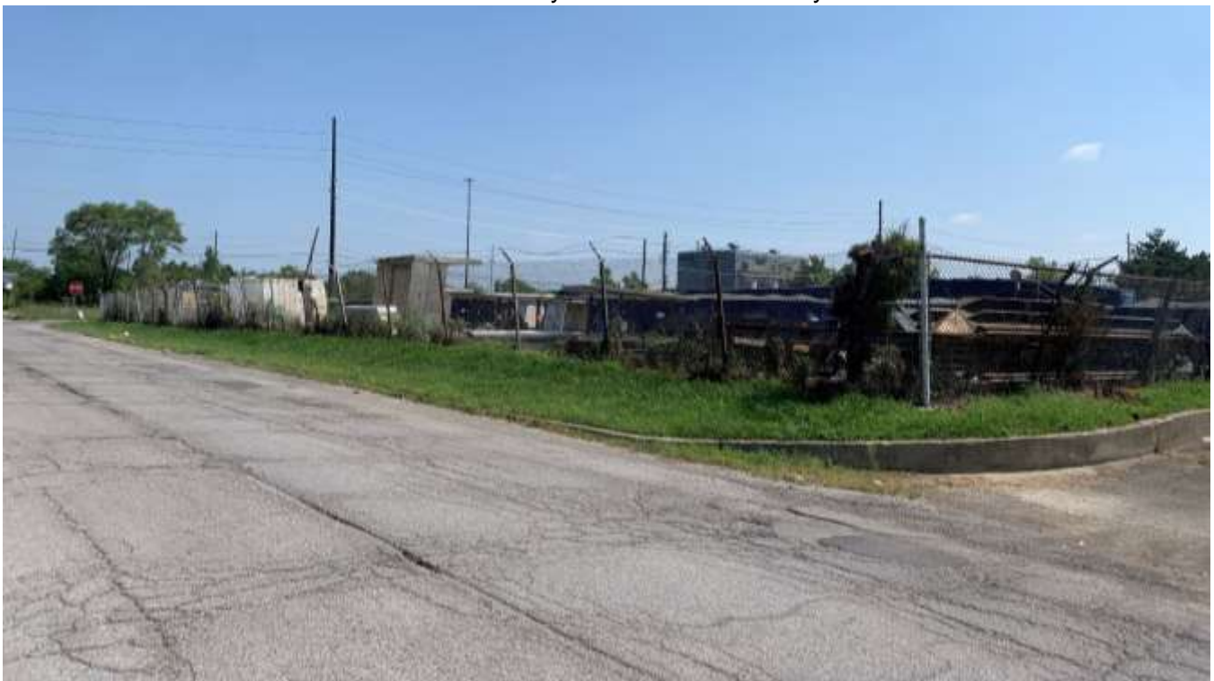
Photo of the subject site street frontage looking north on Olney Street from the closed driveway on site.
