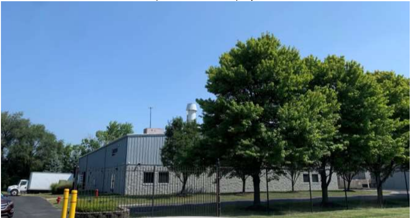
Photo of the pharmaceutical company to the north.
