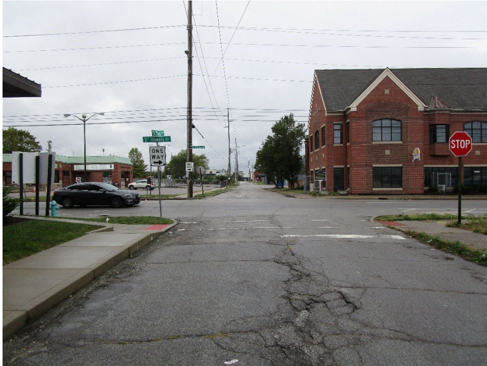
View looking west along Mc Lean Place
