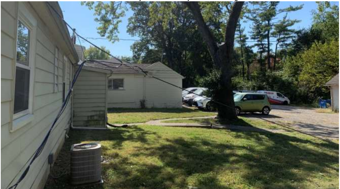
Photo of the rear yard of the subject site looking south.
