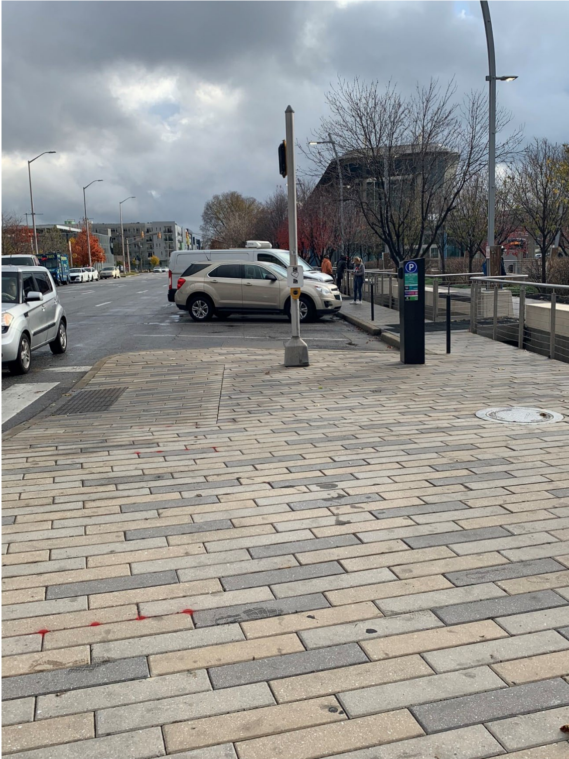
View of existing infrastructure within the Washington Street right-of-way looking east from the Delaware Street intersection
