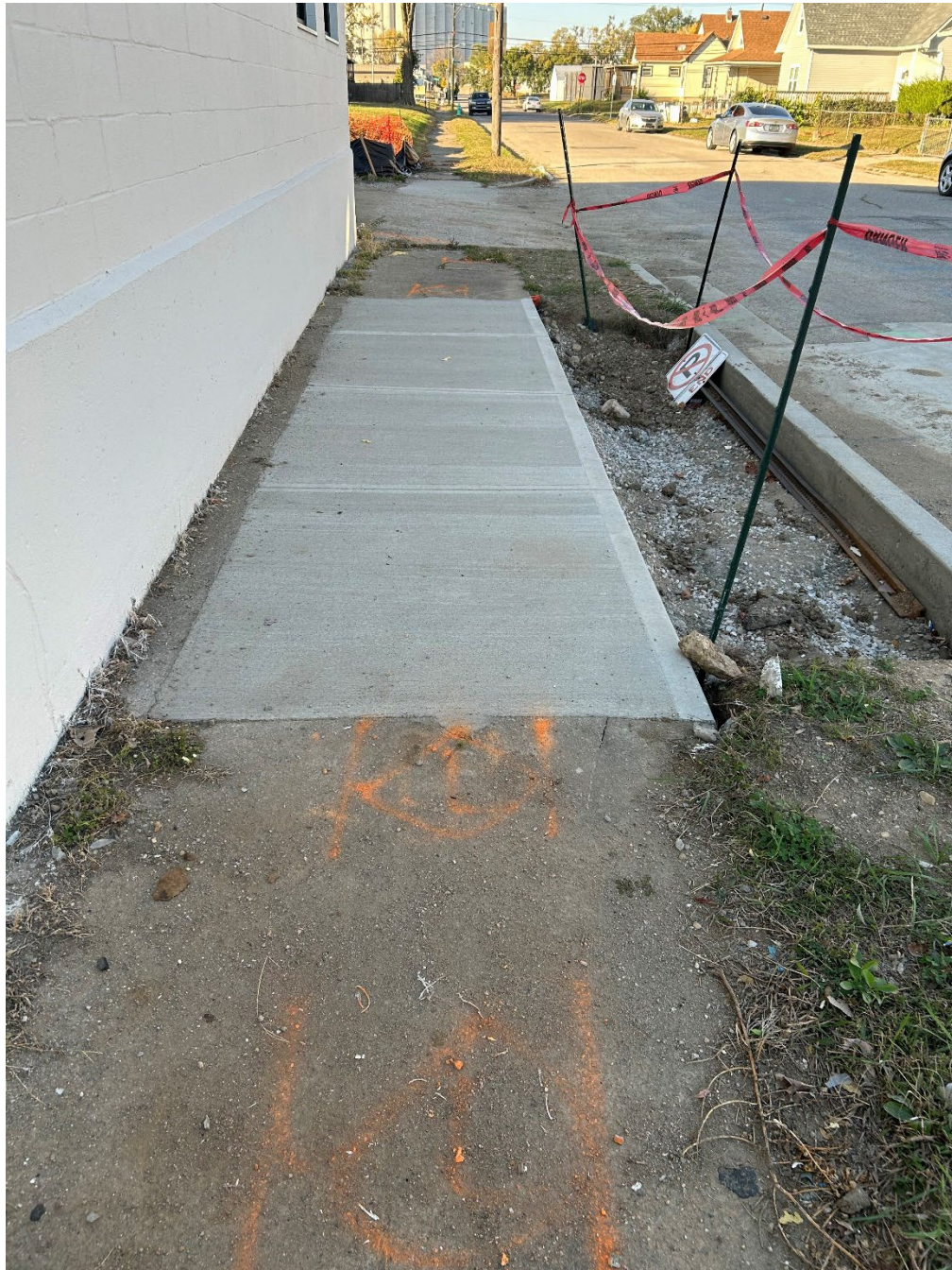
View of existing sidewalk along Rembrandt Street (site is to the left)
