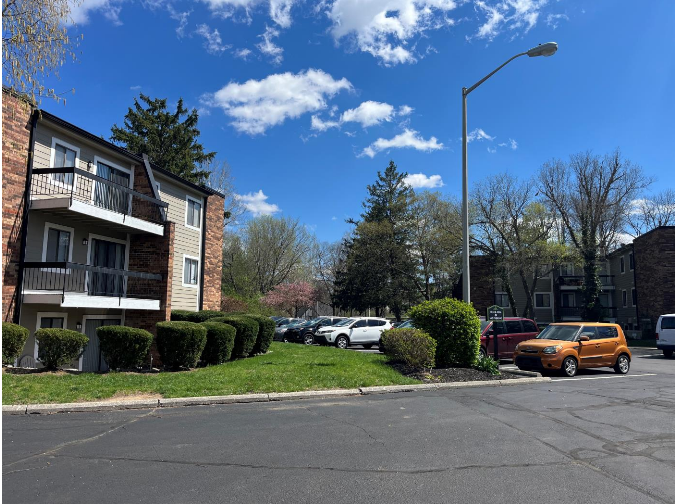
Photo 1: View of apartment complex
