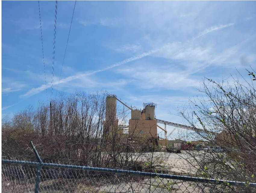
Photo 3: Subject Building Viewed from North
