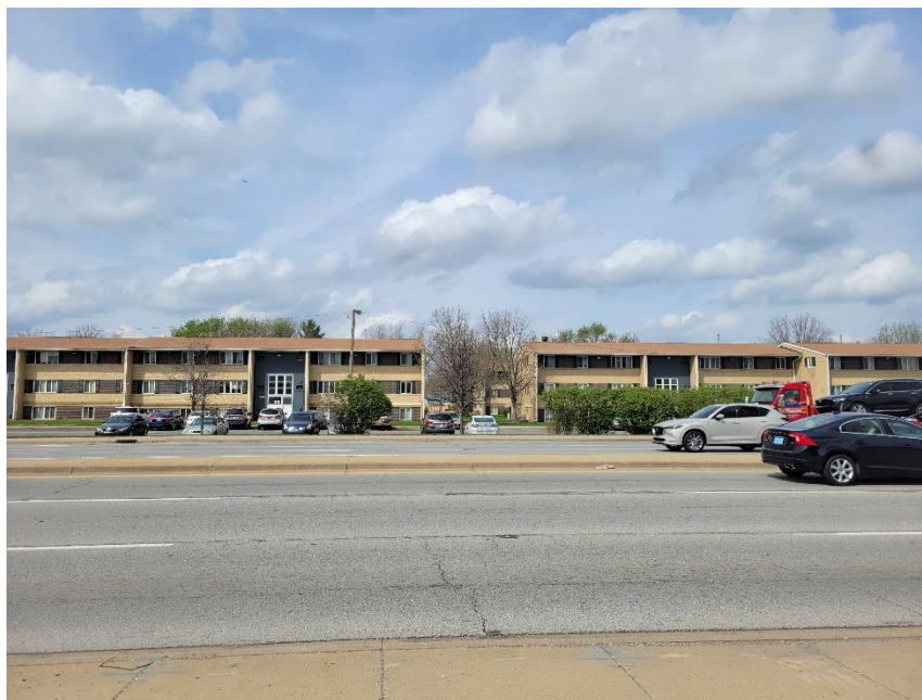
Photo 4: Adjacent Property to North
