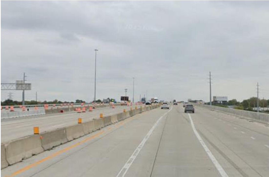
Photo 3: Proposed Billboard Location on Eastern Portion of Subject Site (September 2024)
