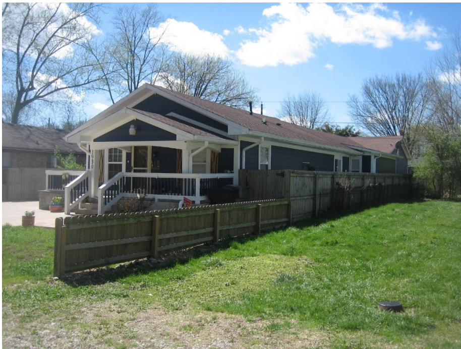
Photo of subject site, north elevation, looking southwest.
