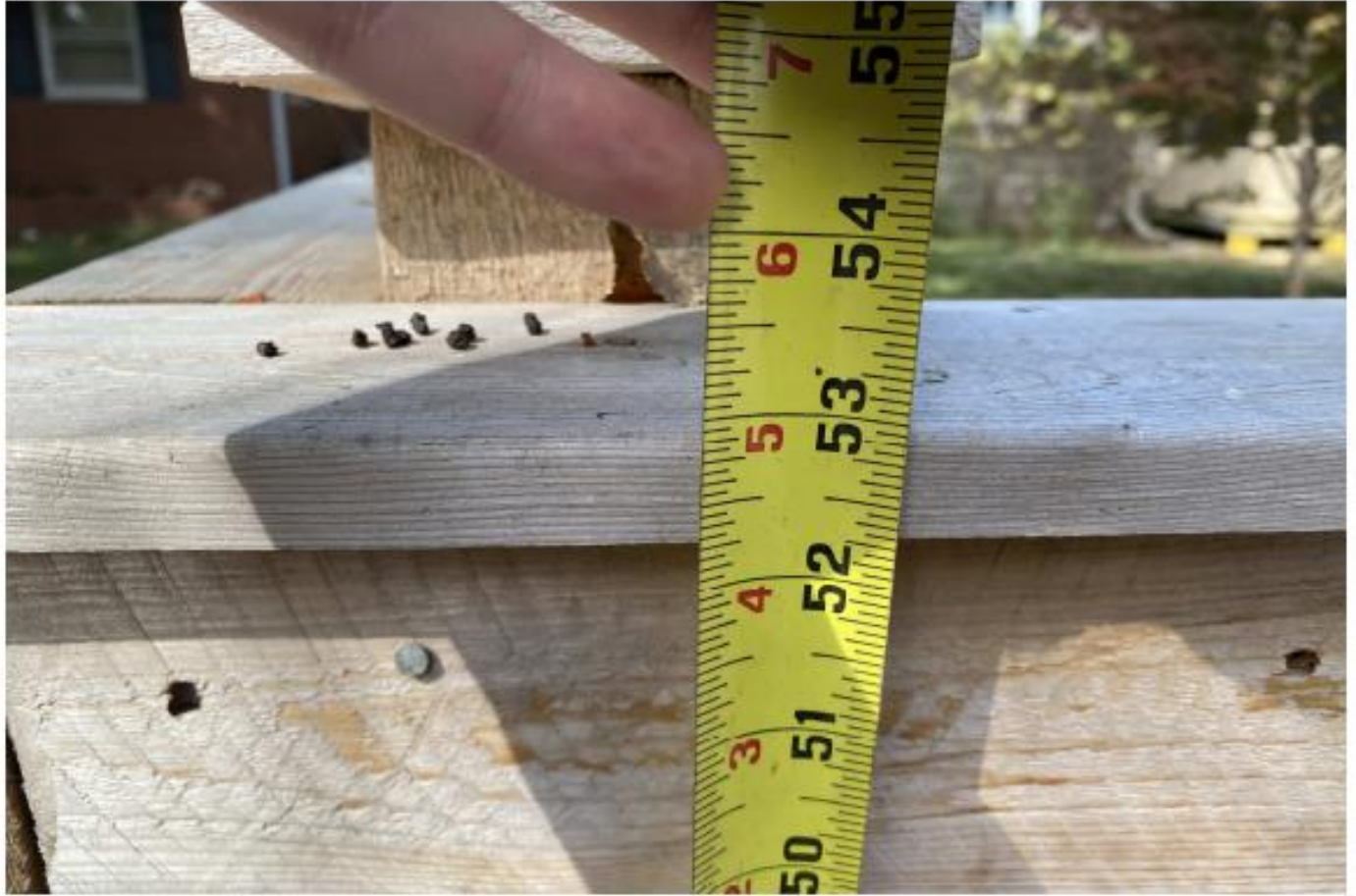
Photo 2: DBNS inspector's measurement of fence height
