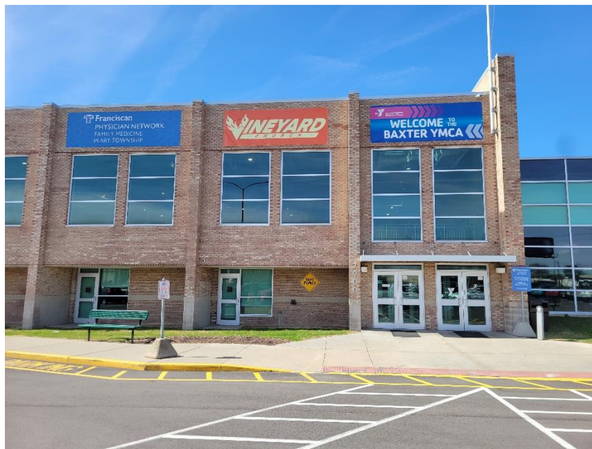
Photo 2: Primary YMCA Entry Viewed from East
