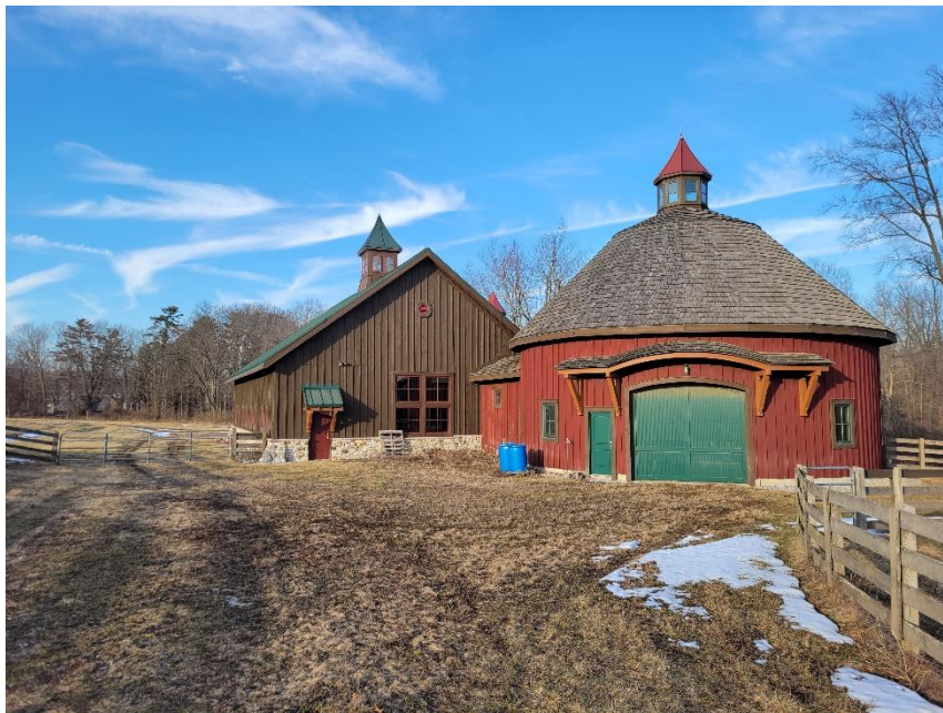
Photo 2: Subject Building Viewed from South
