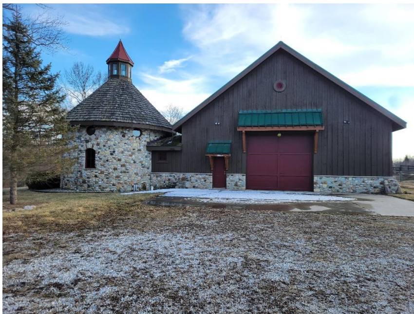
Photo 4: Subject Building Viewed from North
