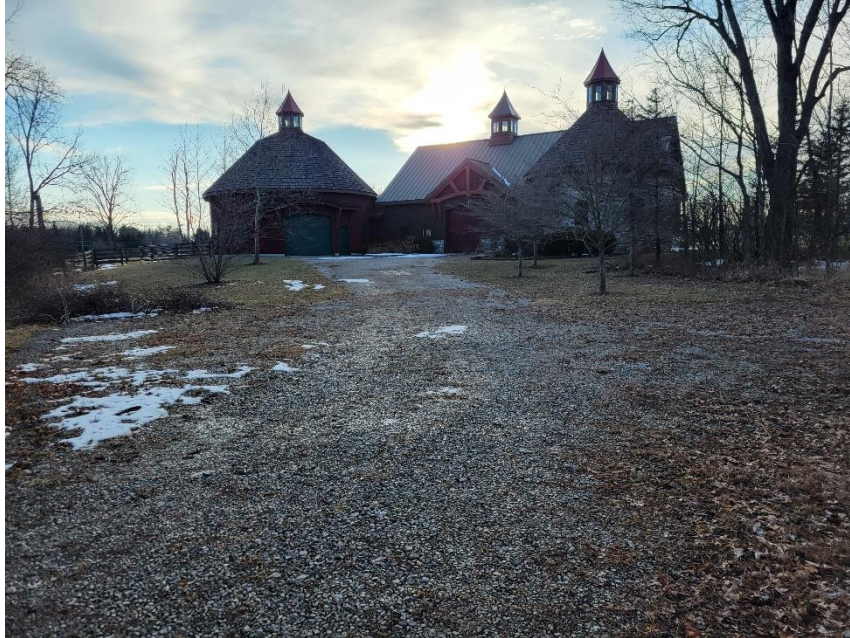
Photo 1: Subject Building Viewed from East
