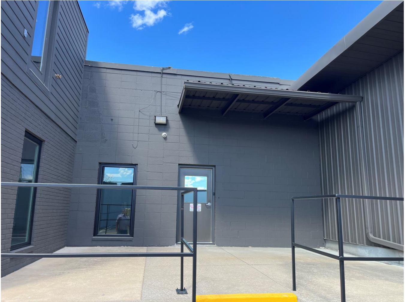
Photo 3: Close-up of area where deck will be installed
