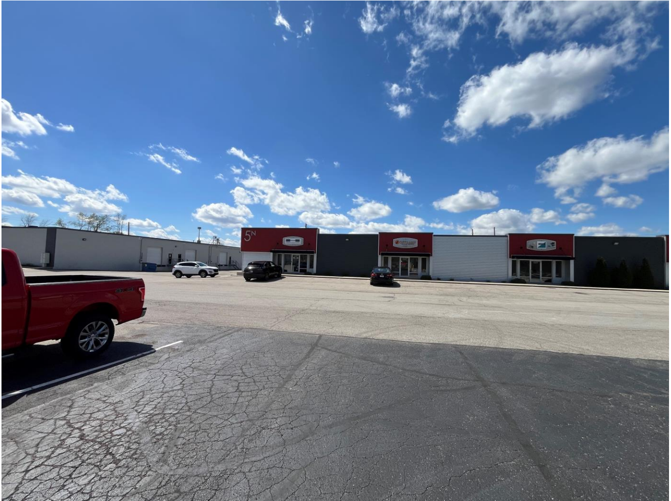
Photo 4: Looking west at neighboring tenant spaces in industrial park
