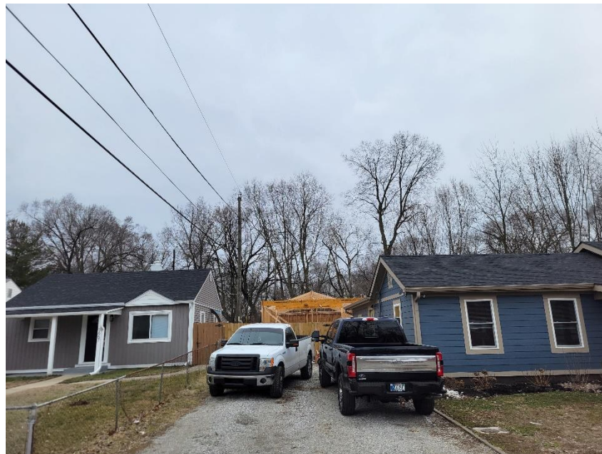
Photo 2: Unpermitted Driveway and Accessory Structure Viewed from North
