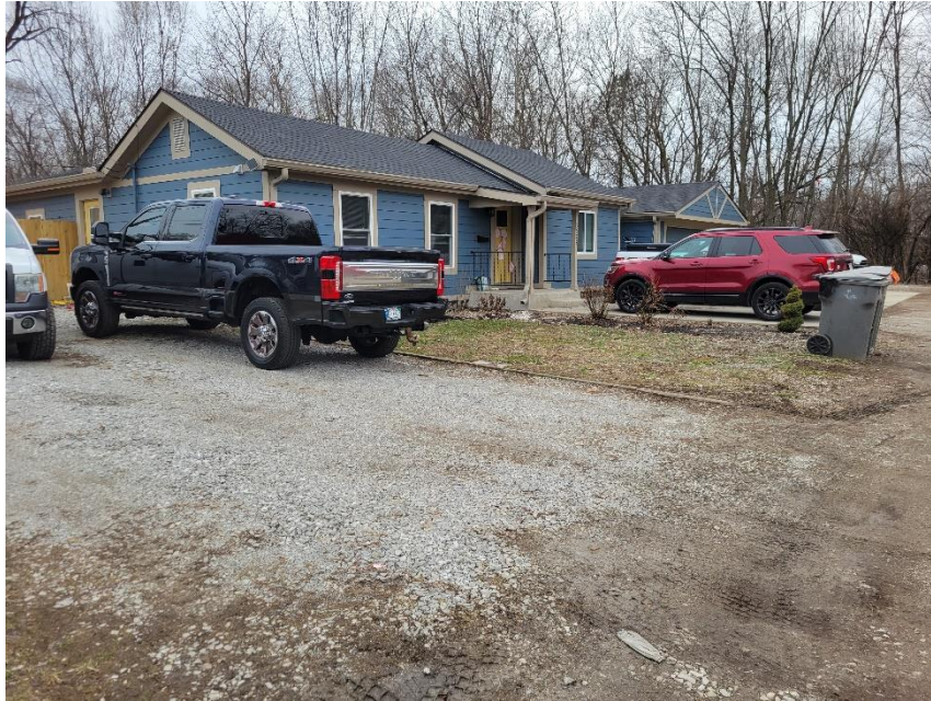
Photo 3: Subject Site Front Yard Viewed from East
