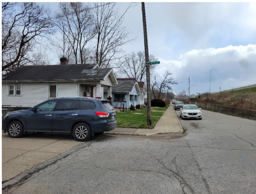
Photo 6: Adjacent Property to South
