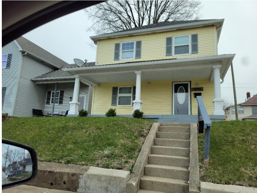
Photo 1: Subject Site Viewed from West
