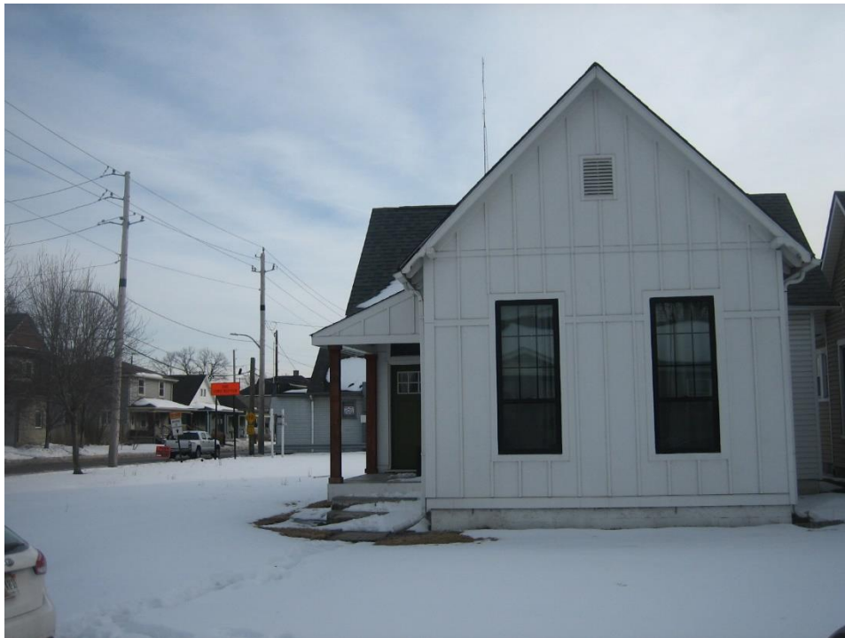
Photo 2 - Adjacent property to the west, looking south.
