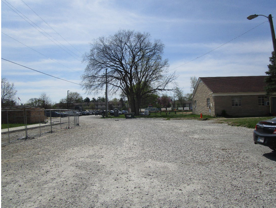
View looking south along northern portion of Haverford Avenue
