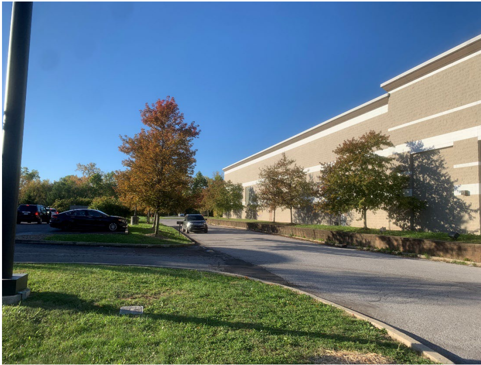
View looking south along western access drive
