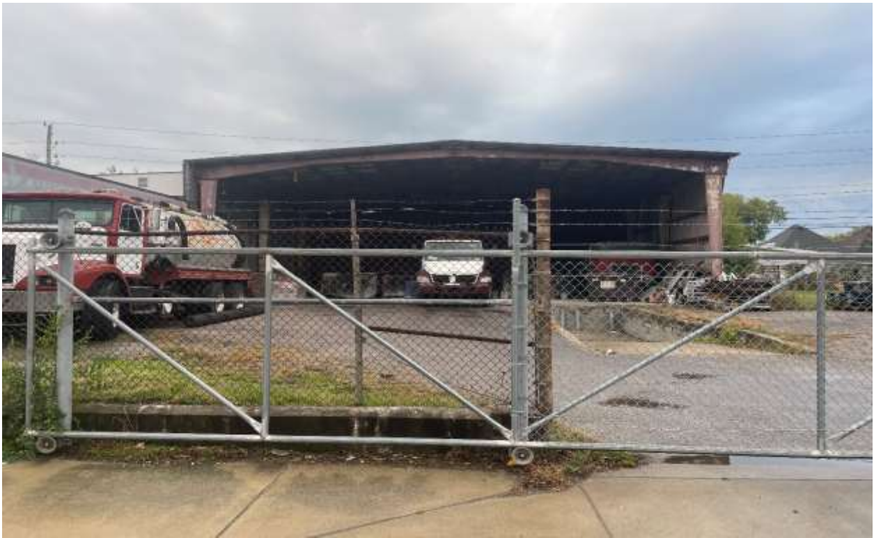
Photo Three: Looking South Towards Subject Site.
