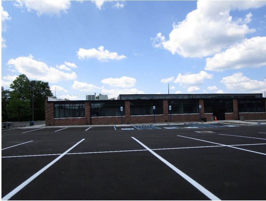
View of the rear of site looking north
