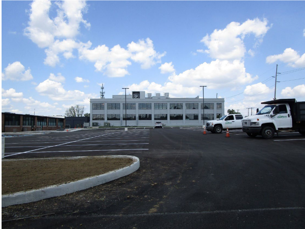
View of the rear of the site looking east
