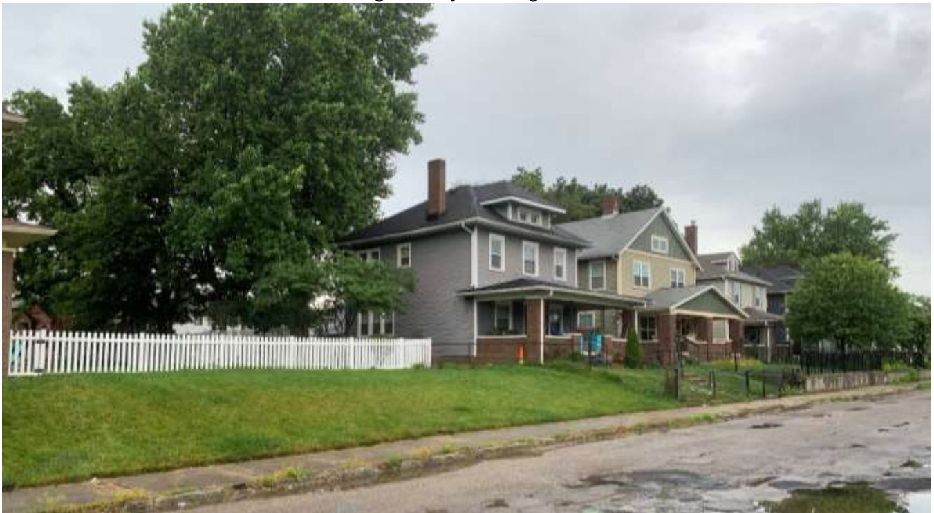
Photo of the single-family dwellings and a two-family dwelling west of the site.
