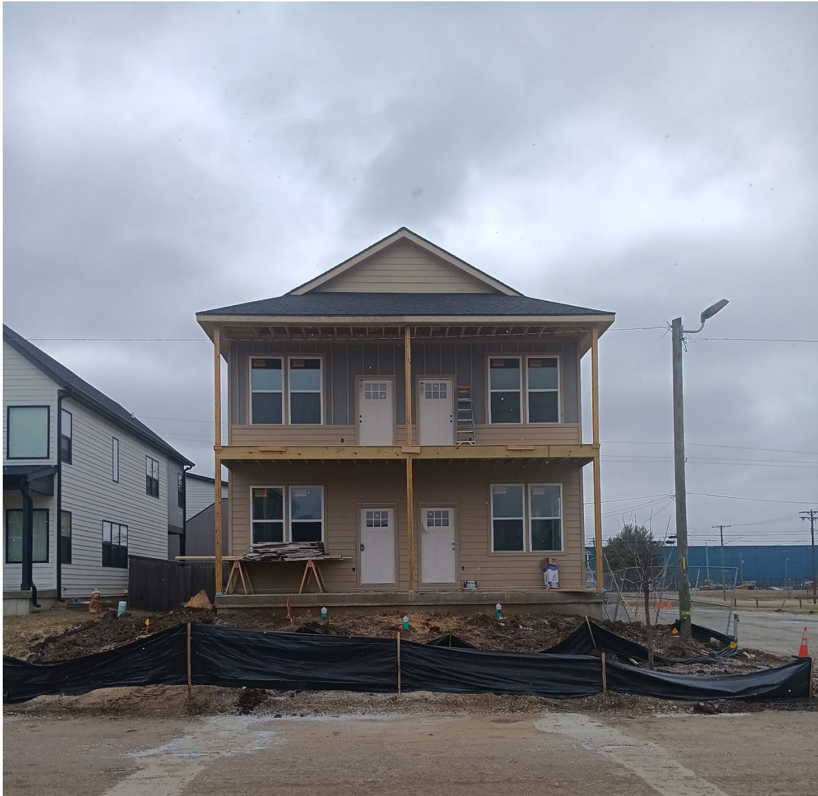
Exhibit 4: Duplex constructed on 2013 Yandes Street.
