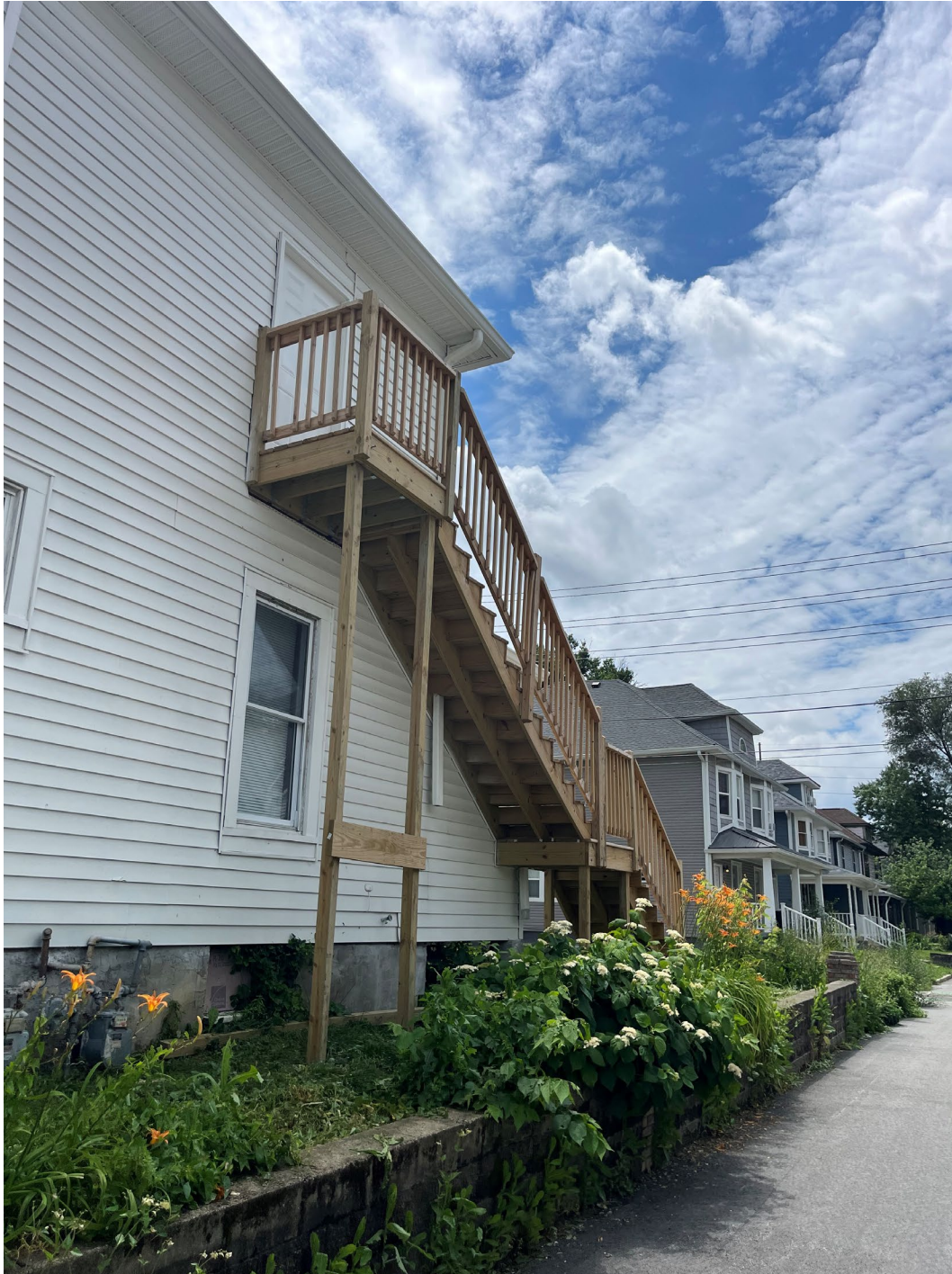
Photo 3: View of stairs seen from multi-use path on New York Street looking west.
