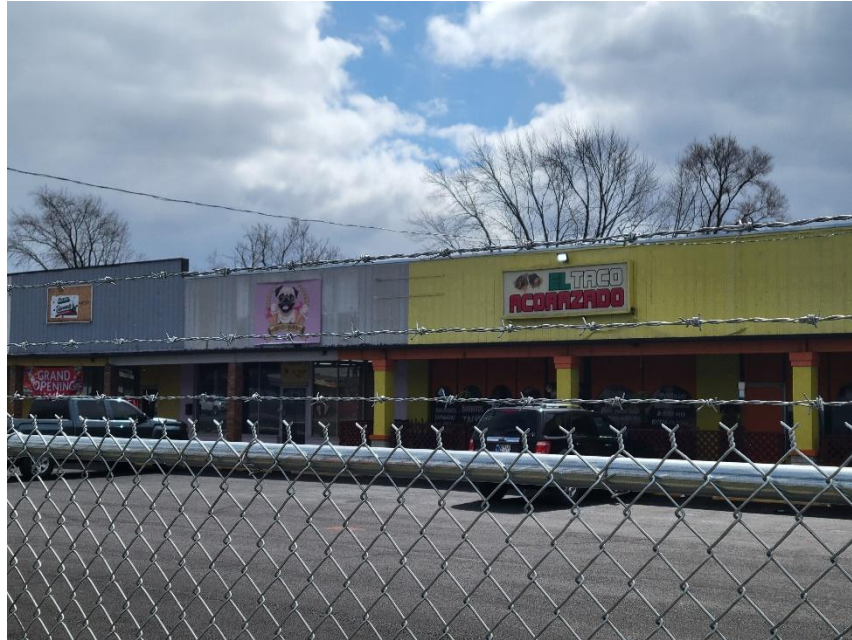
Photo 3: Close-Up of Barbed Wire Fence
