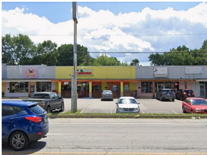
Photo 4: Subject Site Viewed from East (July 2024)
