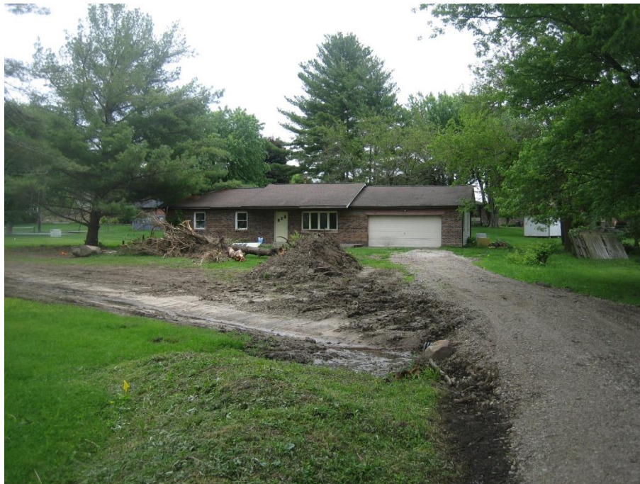
Subject property, existing dwellign to be demolished, looking east.
