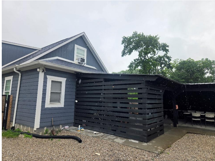
Photo 3: Subject Shelter Viewed from West (Internal to Lot)
