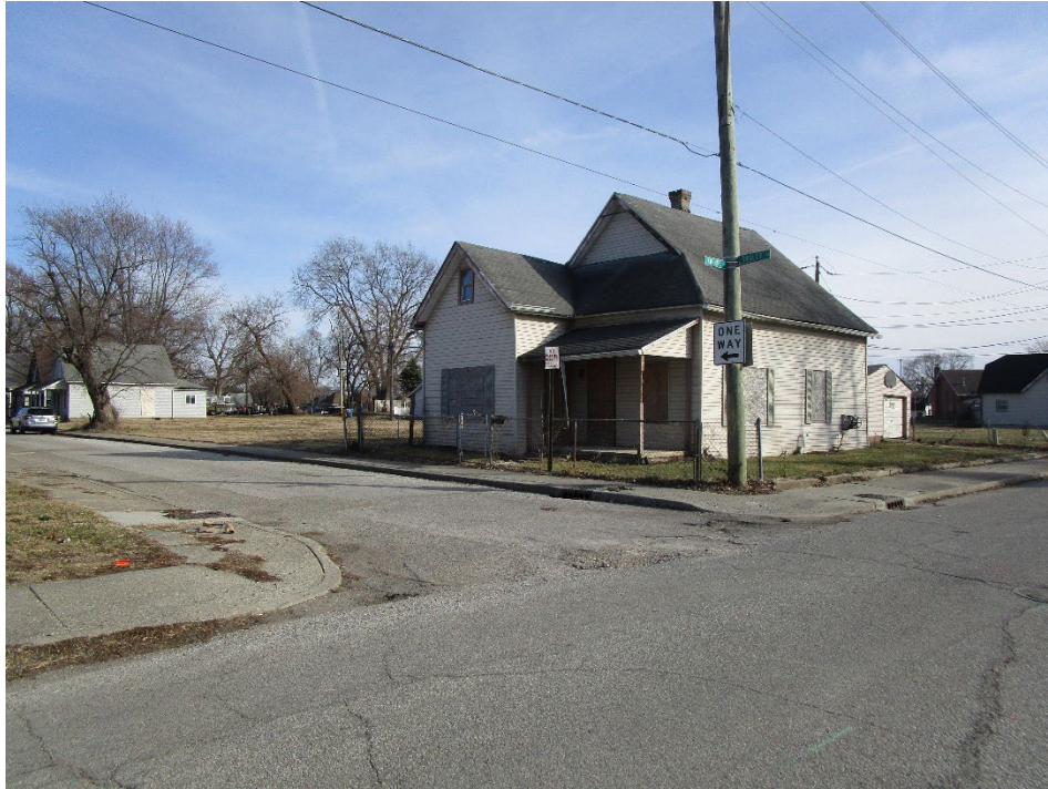
View of site looking southeast across intersection of Koehne Street and Saulcy Street
