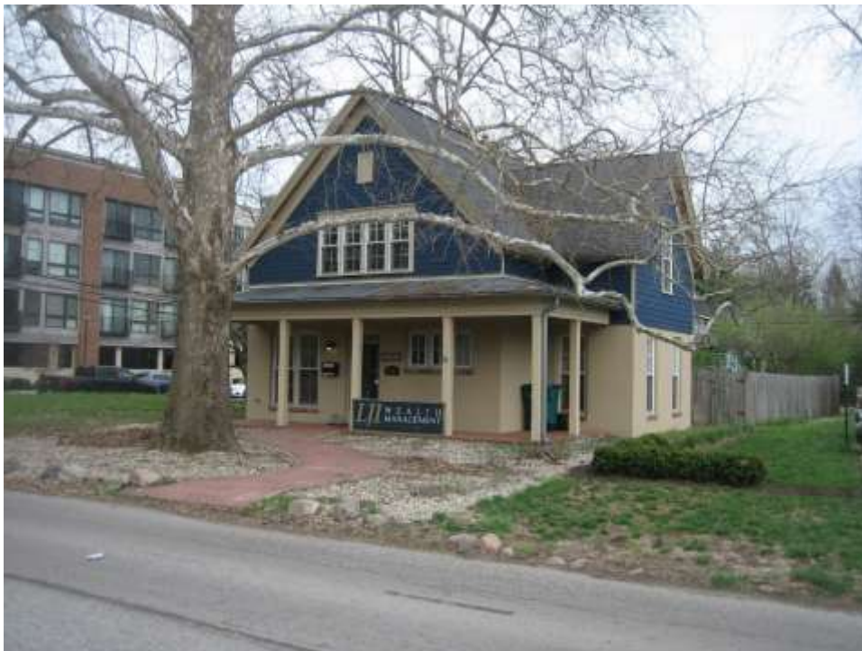
Photo of adjacent commercial office to the north, looking east.
