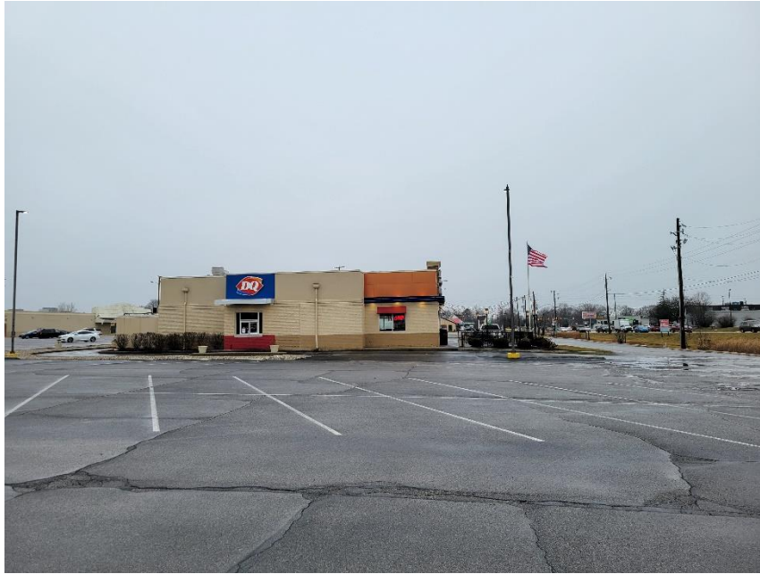
Photo 5: Adjacent Property to the West
