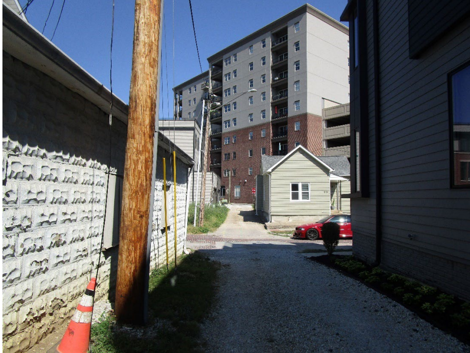
View looking north along north / south alley
