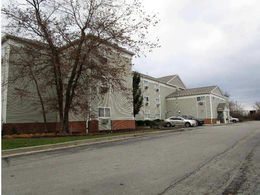
View from site looking northwest at adjacent use to the west
