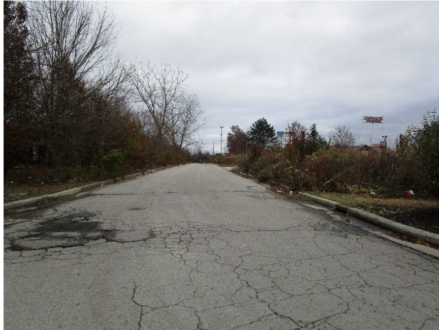
View looking east along Post Drive
