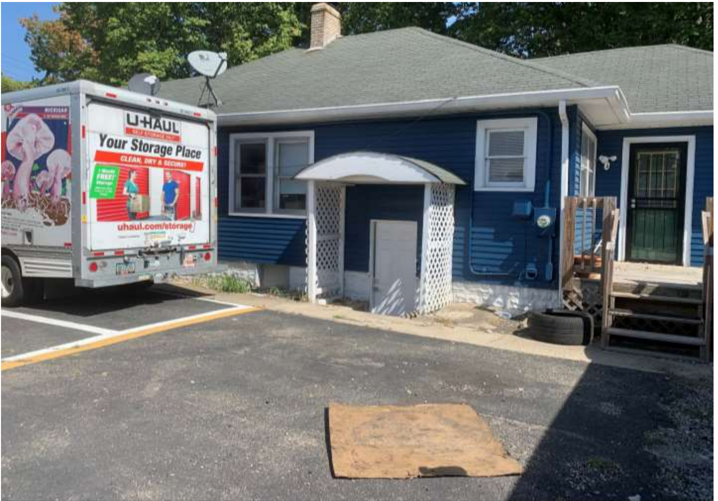
Photo of the western office façade.
