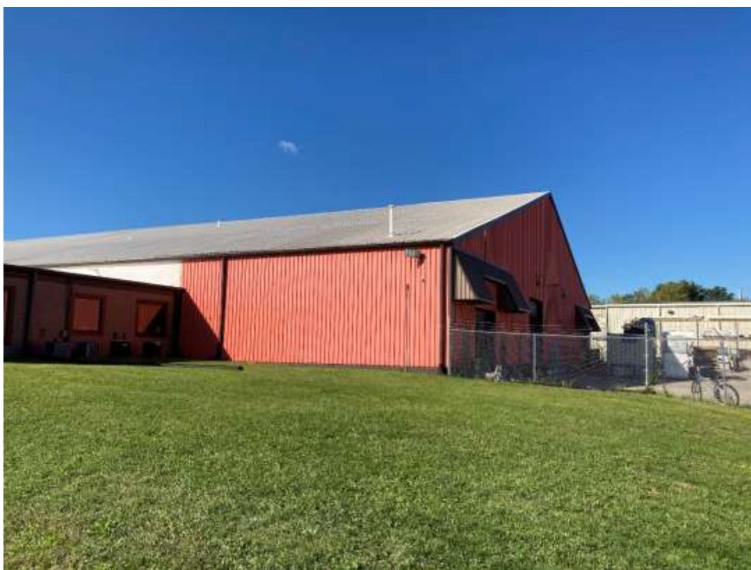
Photo of subject site, with existing structure.
