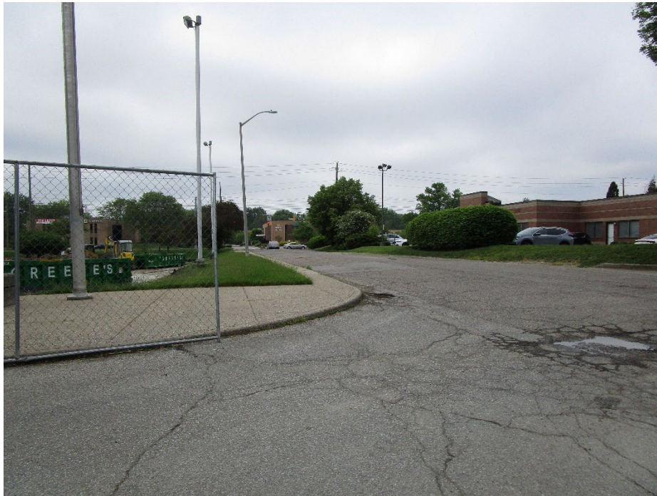
View looking south along Guildford Avenue
