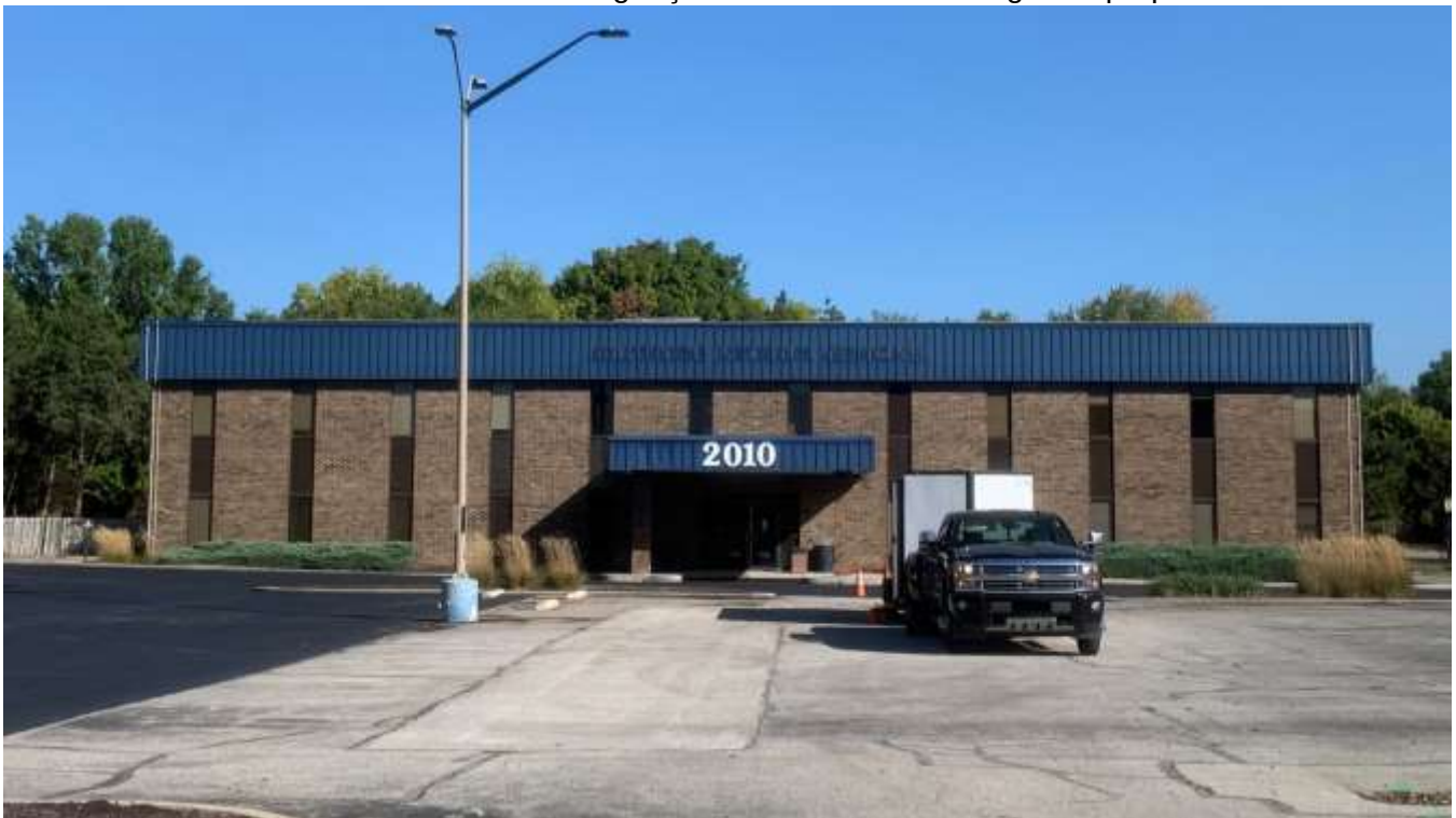
Southern building façade where new wall sign is proposed.
