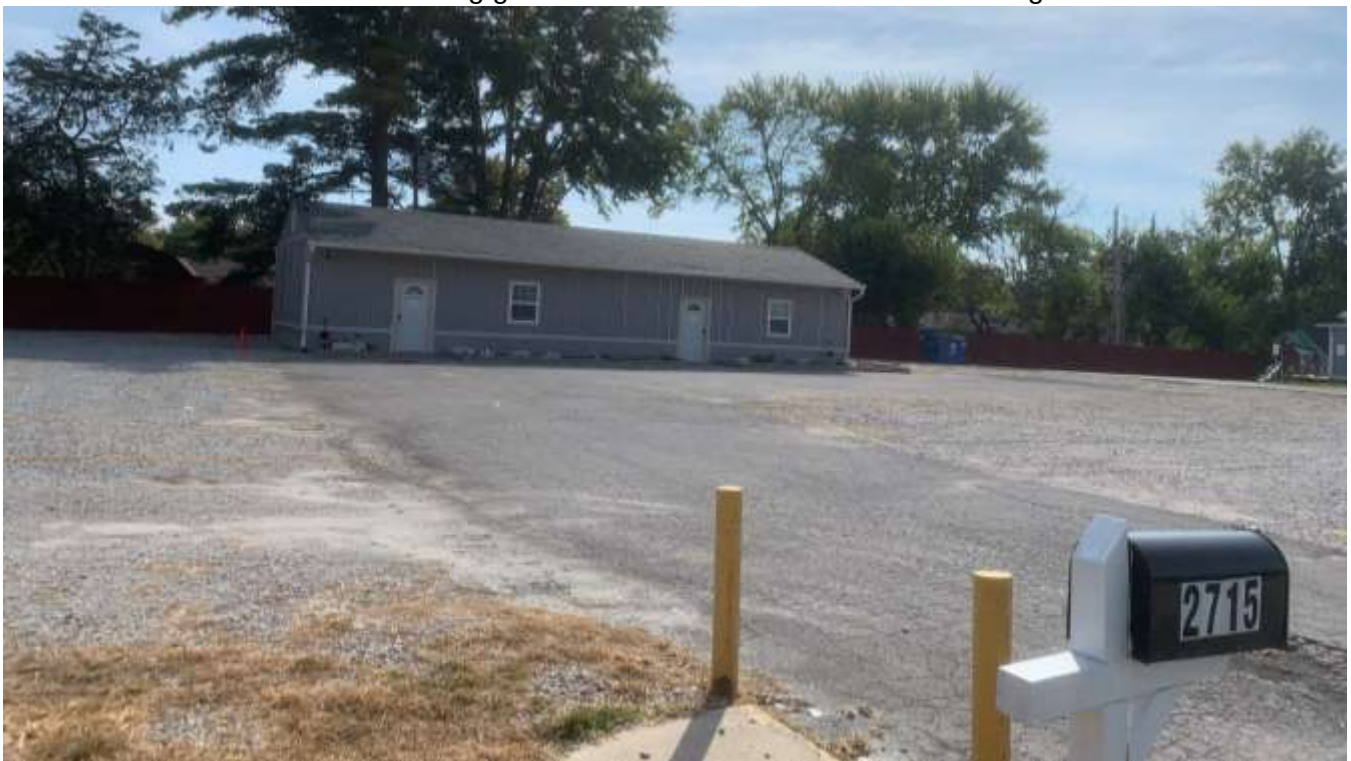
Photo of the existing building on site at 2715 North Post Road.
