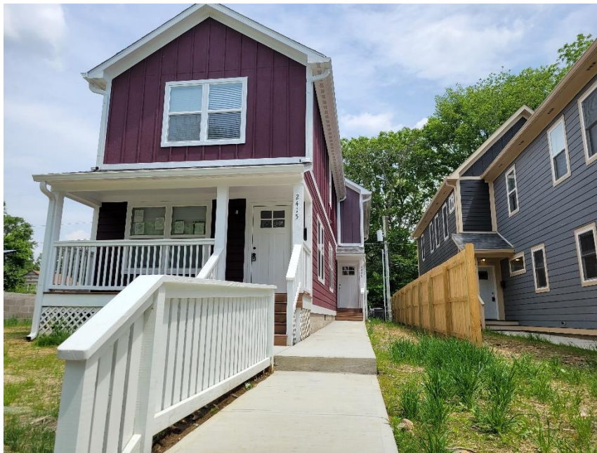
Photo 2: 2415/2417 N Rural Viewed from West
