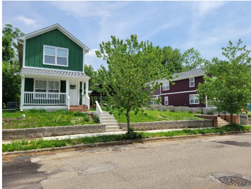
Photo 5: Both Structures Viewed from West
