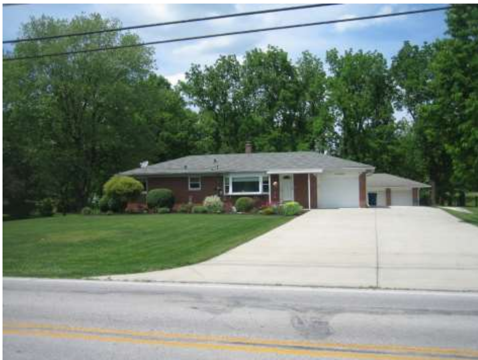
Adjacent single family dwelling to the north
