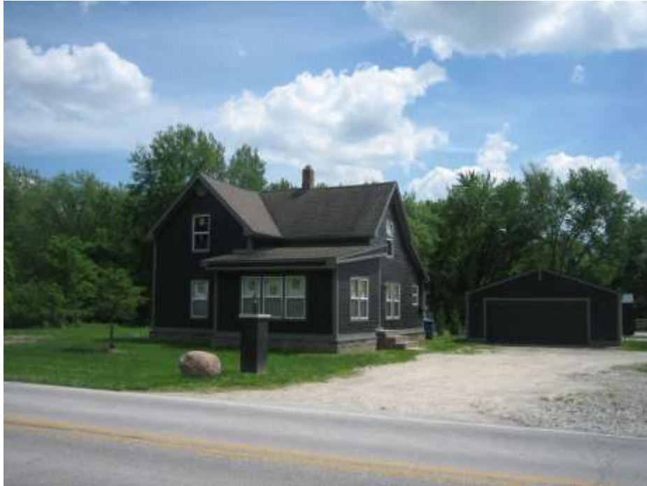
Subject site single family dwelling, looking southeast
