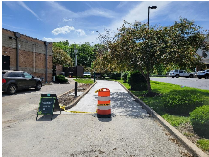
Photo 6: Beginning of Drive Lane viewed from East
