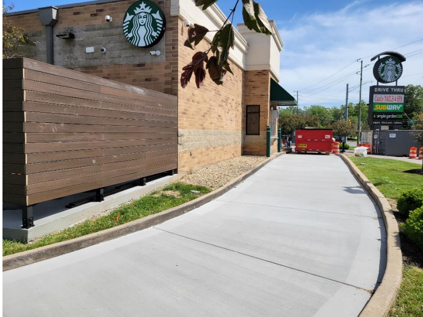
Photo 3: End of Drive Lane viewed from North
