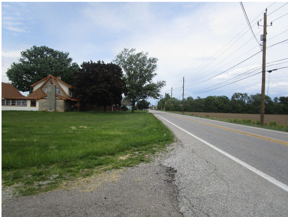
View looking north along Bluff Road
