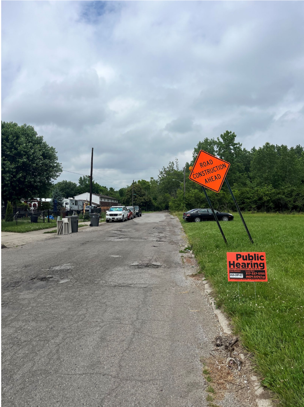
Photo 4: Wagner Street looking north
