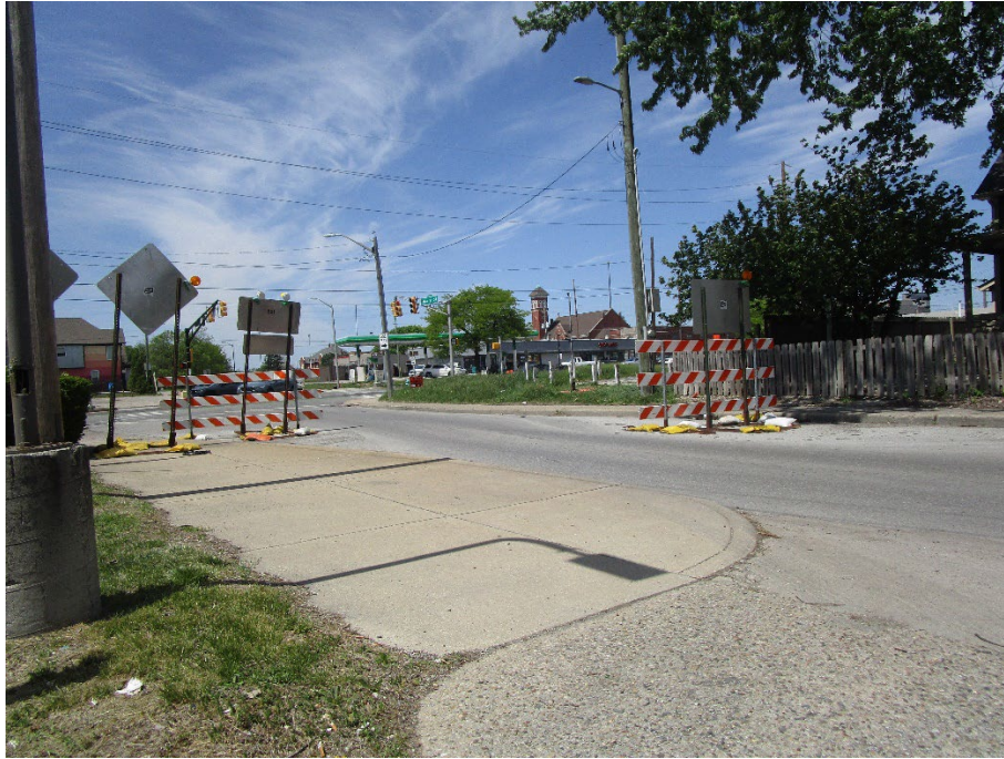
View of site looking northwest across East Morris Street
