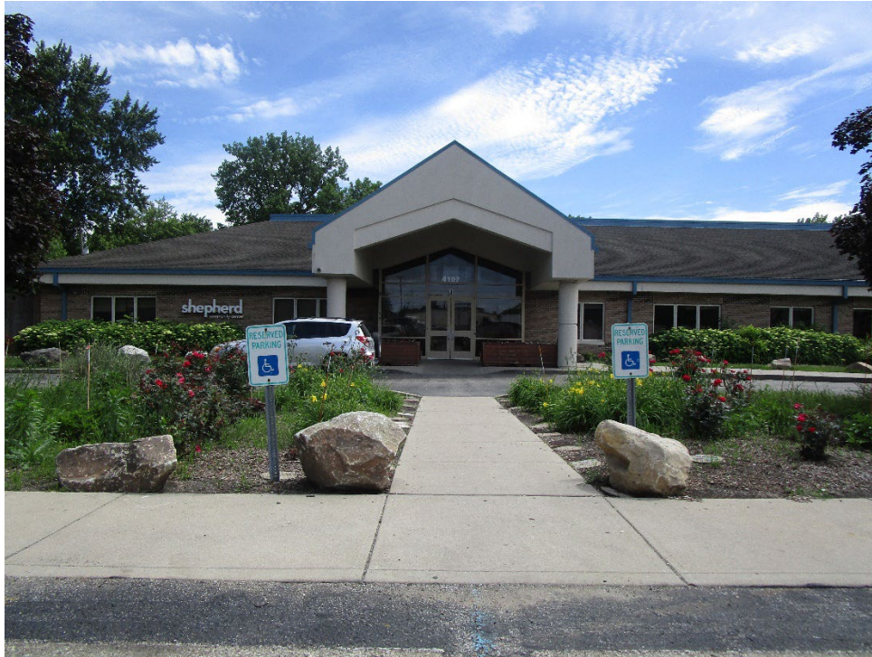
View of Community Center looking south
