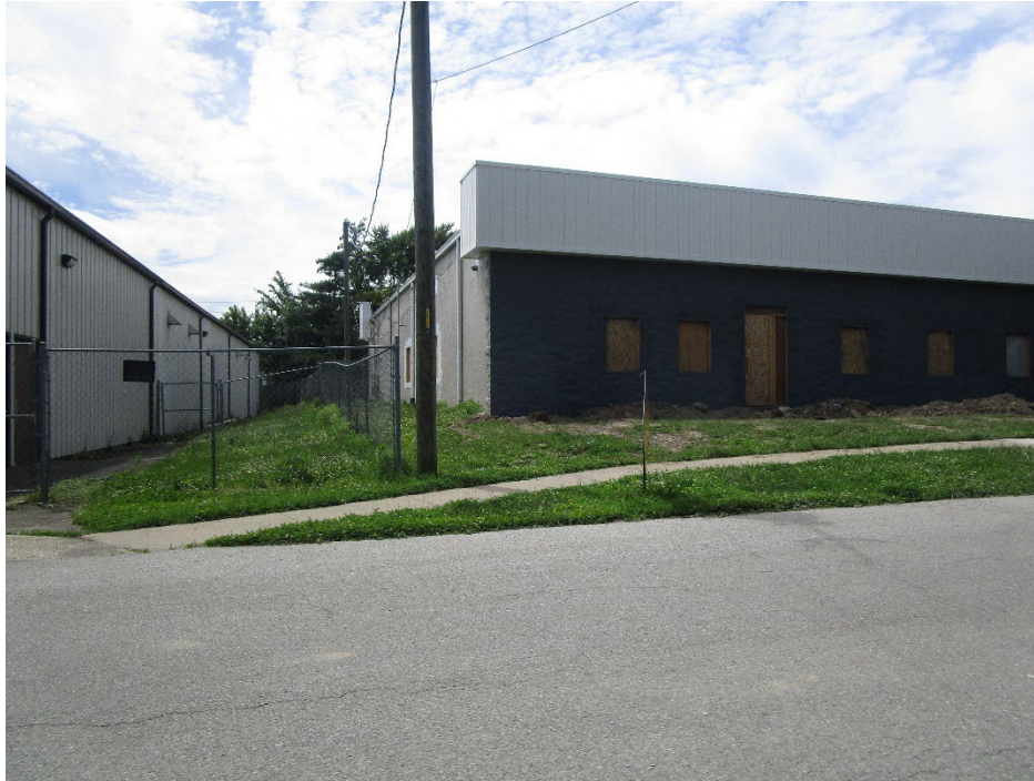
View from access drive looking west at commercial building (the Porch)
