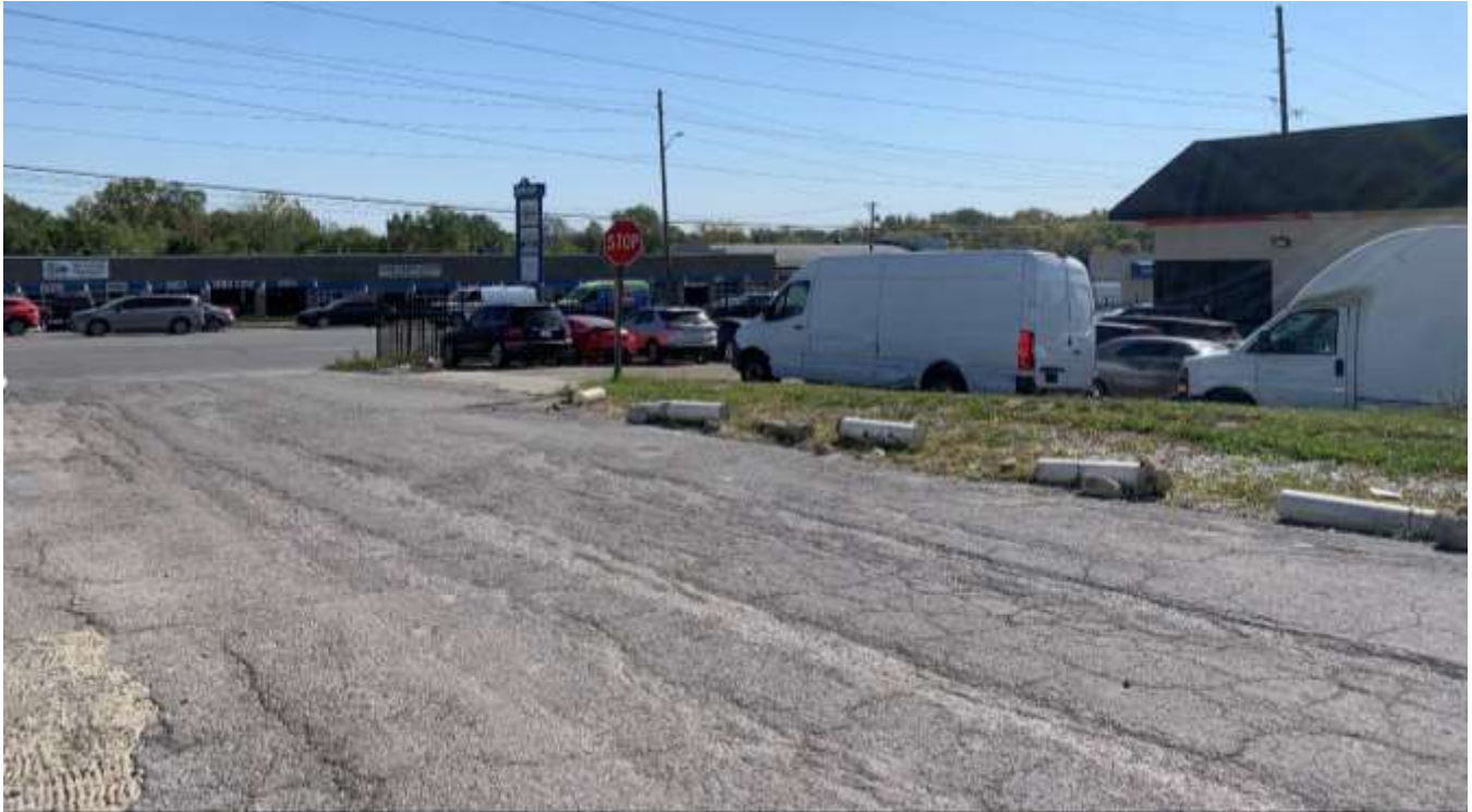
Photo of the subject site looking southeast from 45 th Street.
