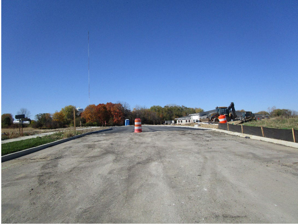
View looking west along private drive
