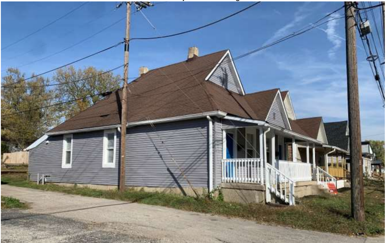
Photo of the subject site looking east.
