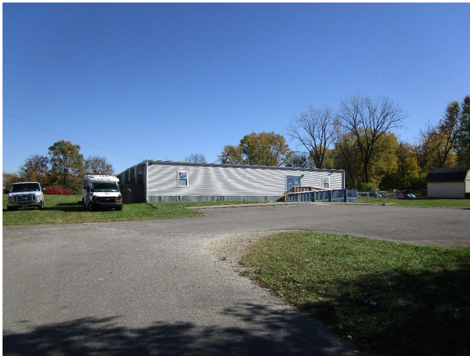
View of site looking southeast
