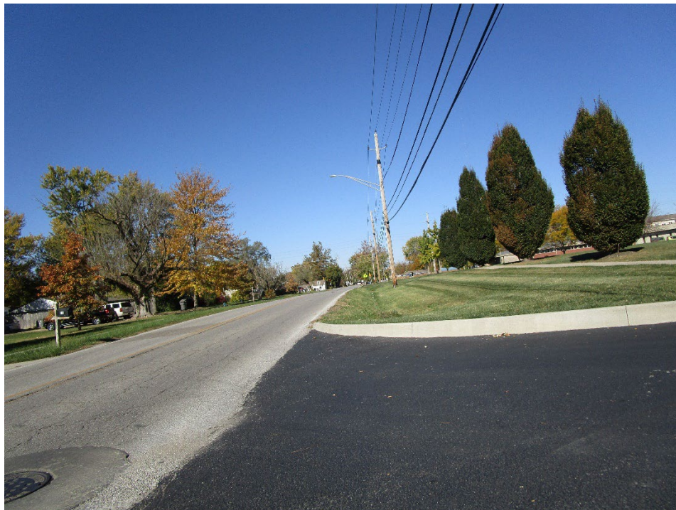
View looking north along North Ritter Avenue
