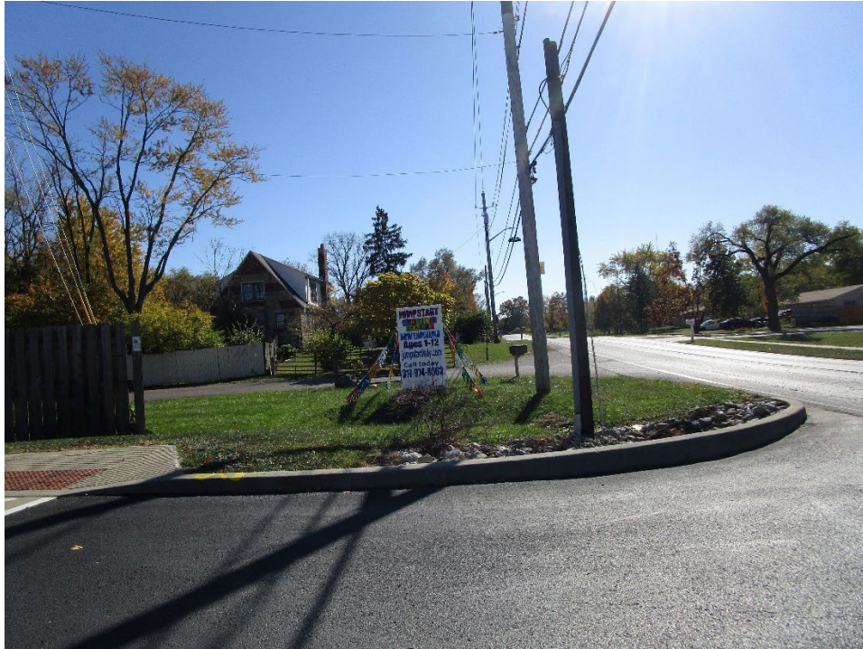
View of site entrance drive looking south
