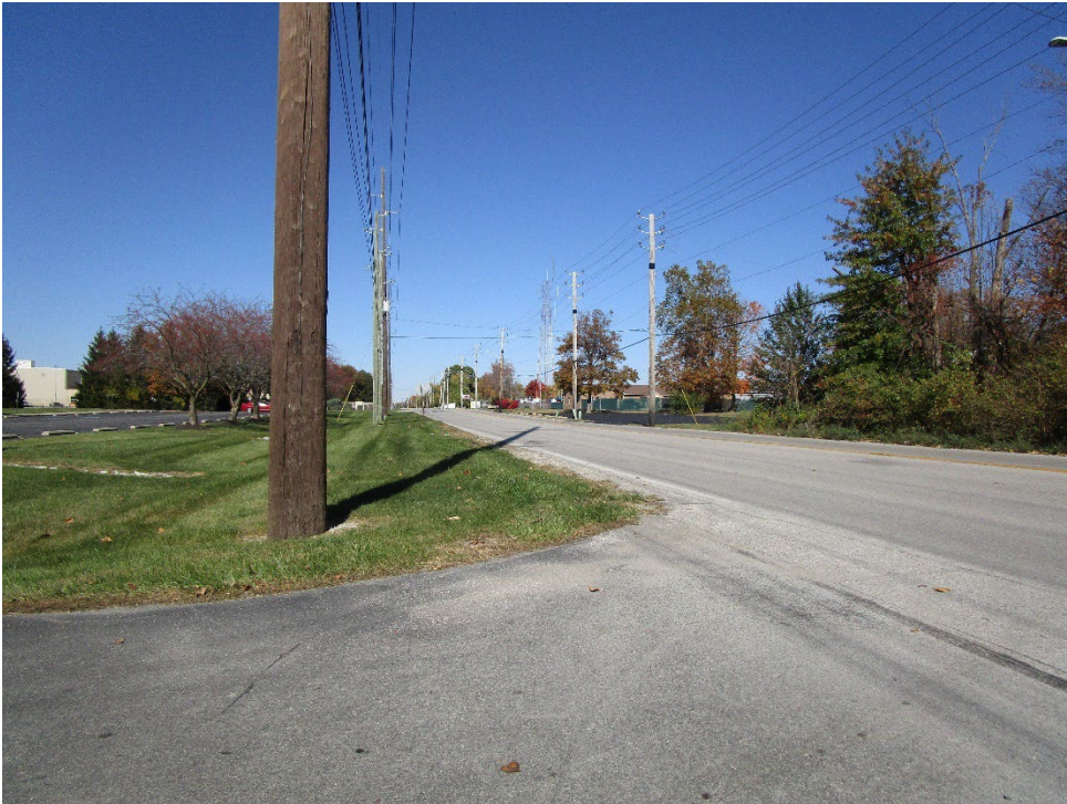
View looking north along South Shortridge Road
