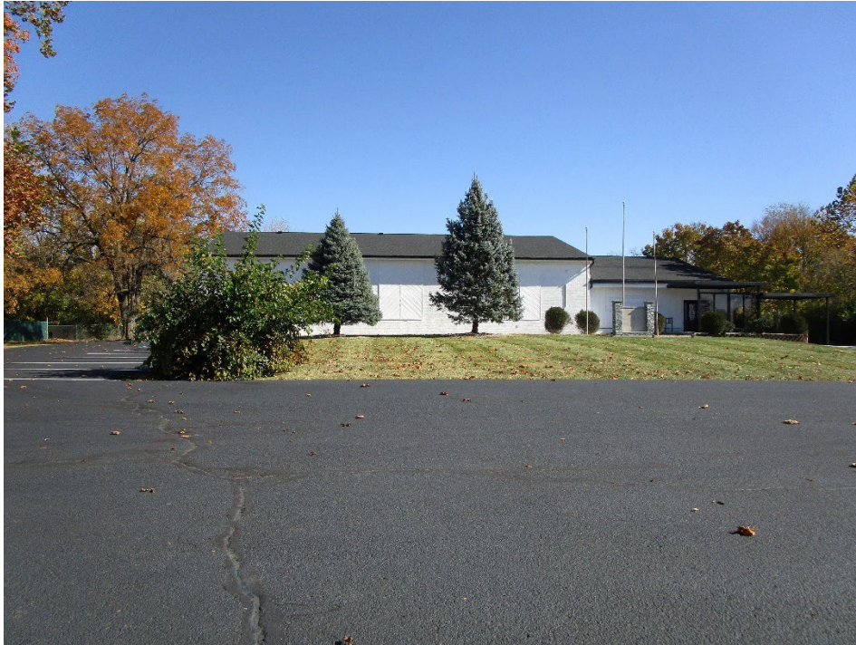
View of site looking east
