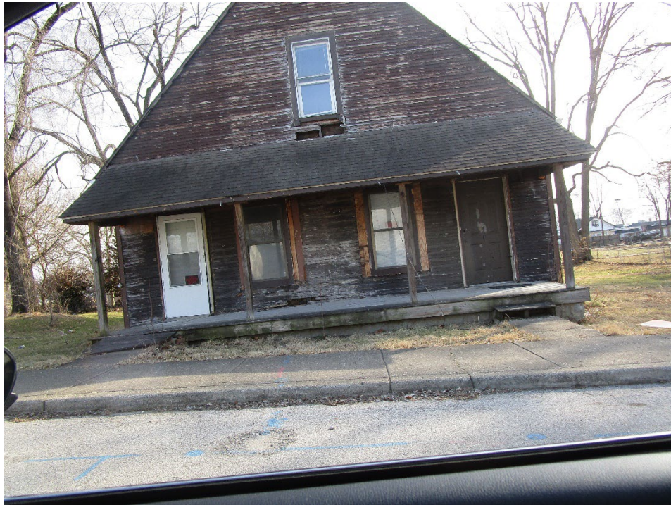
View of site looking south across Saulcy Street
